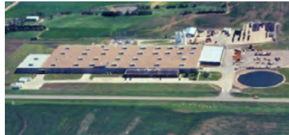
Hoisington Communications Plant | Hoisington, KS
