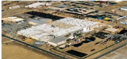
Brownwood Communications Plant | Brownwood, TX
