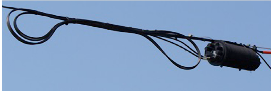
Example: 3-Loop Retrofit Without Storage Devices
